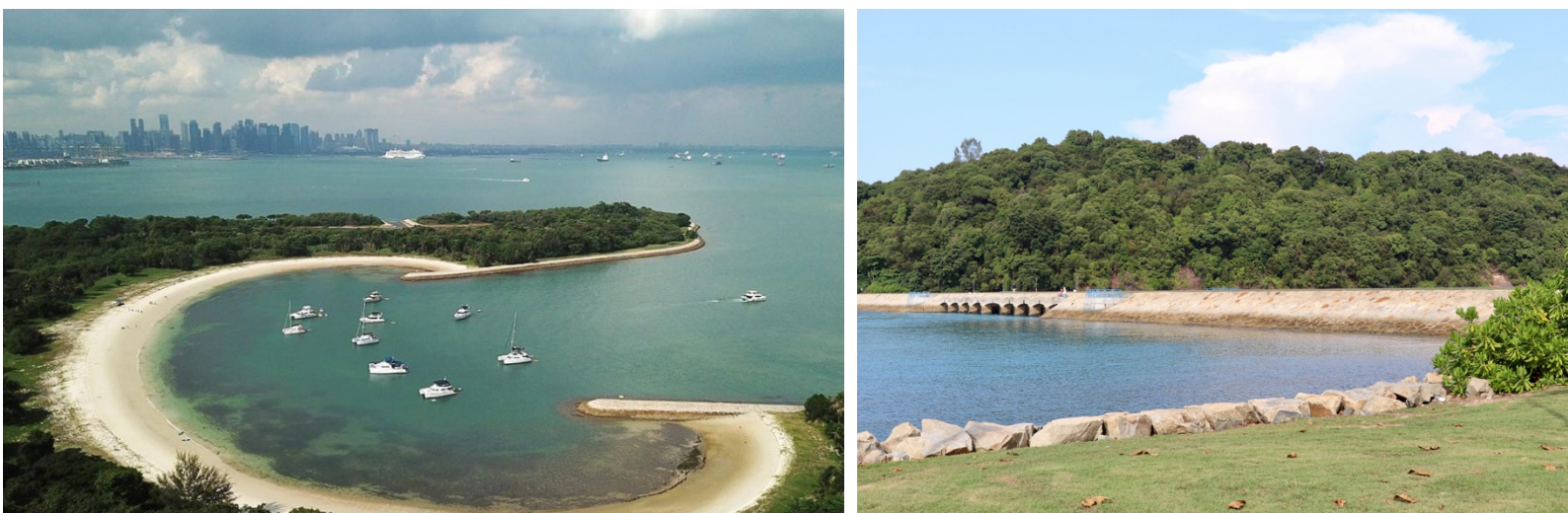
Figure 6 Major developments to the SJI-C. (Left) Eagle Bay constructed on the new Lazarus Island (now including Pulau Seringat and Kias). (Right) Causeway that connects St. John's Island and Lazarus Island constructed. Photos by Lee (2019) and Rachel Oh.
