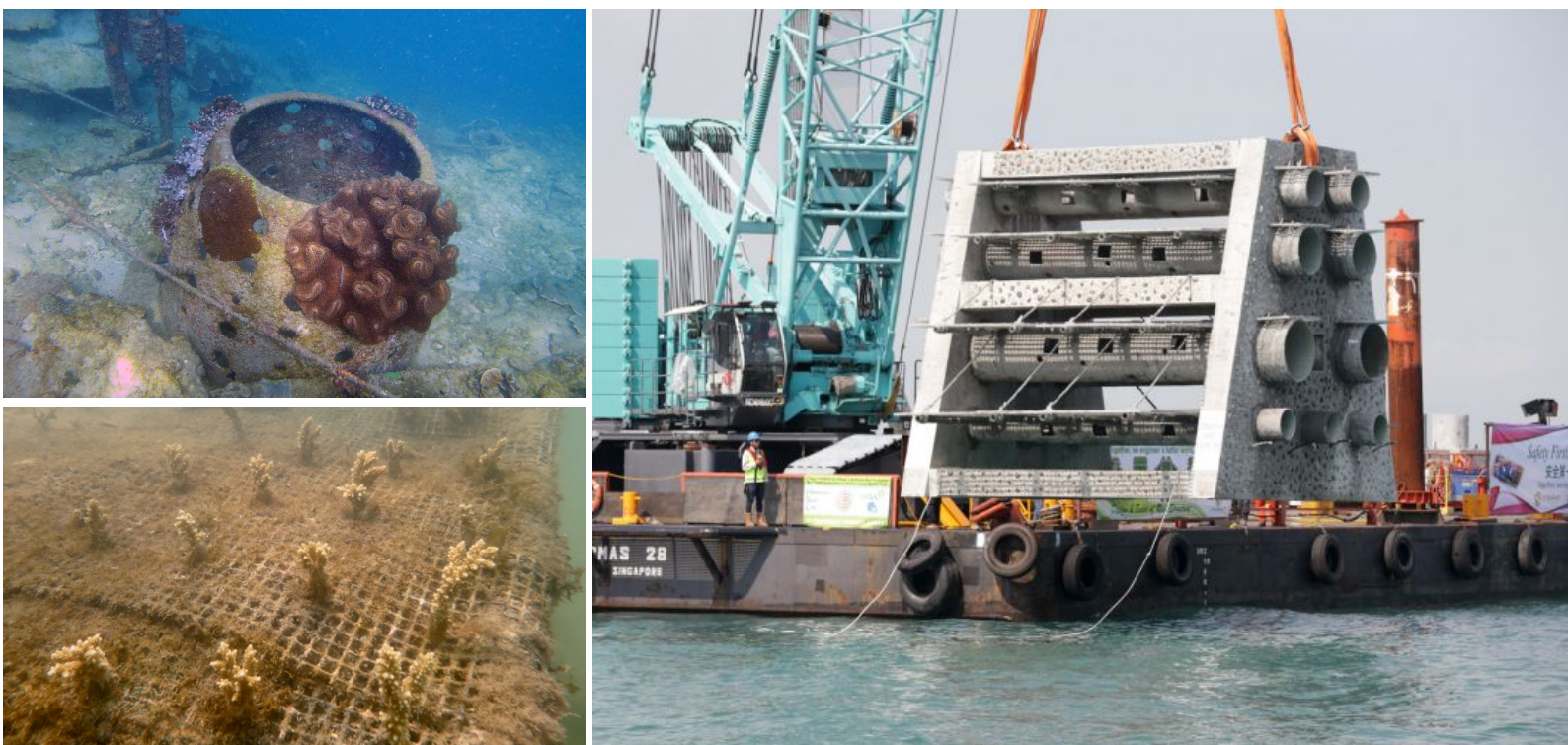
Figure 43 Reef restoration projects carried out in the Southern Islands. (Top left) Reef Enhancement Units (REUs) with coral recruitment. (Bottom left) Coral fragments propagated in coral nurseries to be transplanted onto subtidal seawall. (Right) Singapore's largest reef structure being installed at the Sisters' Islands. Photos by Reef Ecology Lab and Ng (2019).
